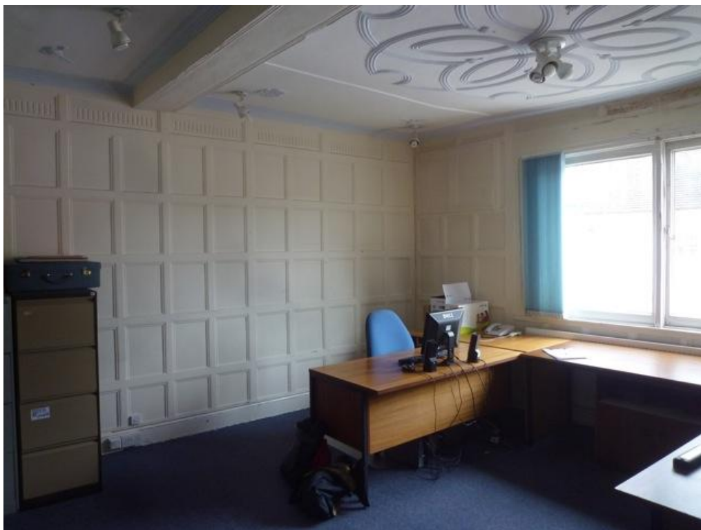
The room is lined with small-square panelling, five panels high with a frieze. It has been very little altered.
