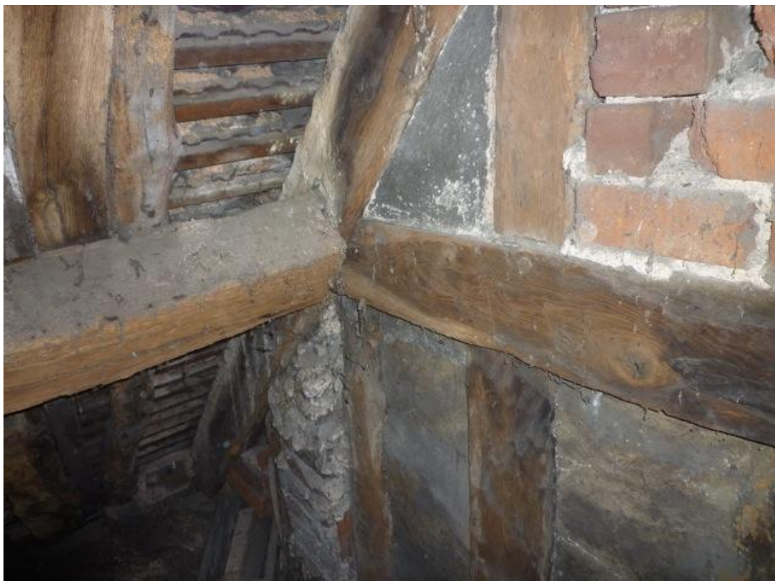
Detail of tenoned purlin set in gable of south-east wing
