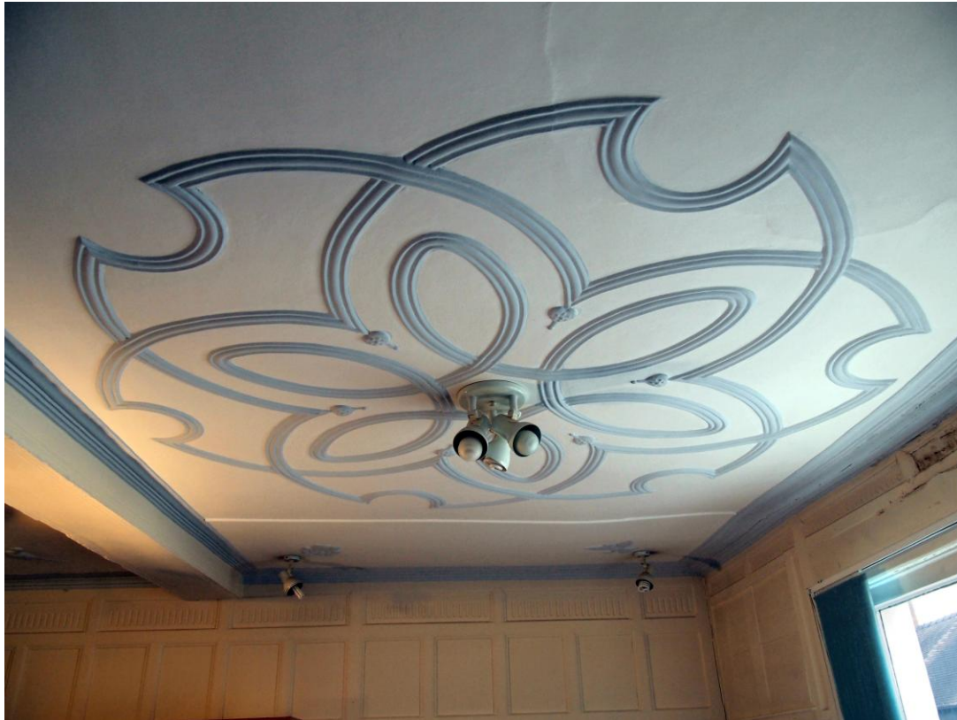
Plasterwork of the ceiling panel closest to the street. (Paul Jones LRPS)
