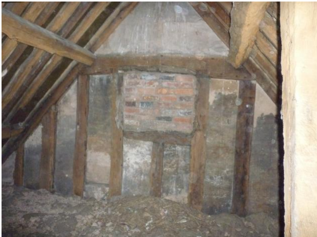
Top: roof space of the main range looking west with a blocked window in the end gable. Bottom: roof space of main range looking east with another blocked window.
