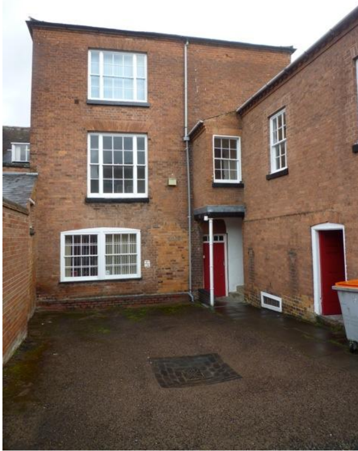
South or rear elevation showing on the right the brick wing. The porch roof is supported by the elegant cast-iron Victorian Gothic clustered column. The datestone (fig p33 below) is set in the room on the right through the open door.
