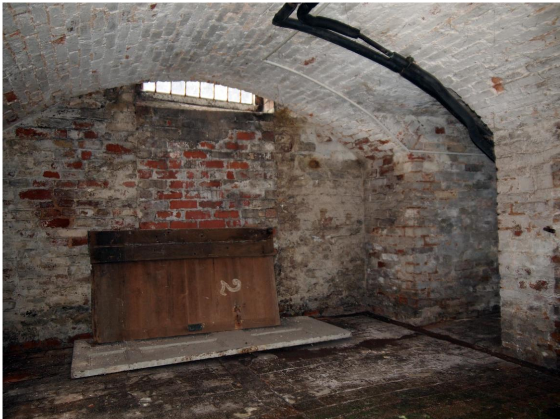
The cellar under the north-east rear wing has a barrel vault and although showing some stonework at its lowest level does not appear to be any earlier than c.1800. (Paul Jones LRPS)
