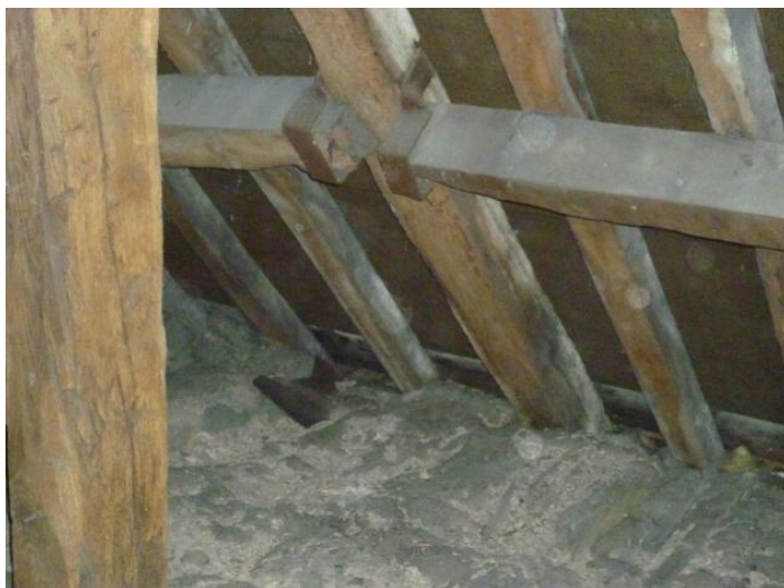
Details showing the iron straps used to hold the lower tier of purlins to the principal rafter of the intermediate truss.
