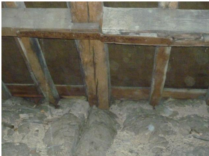
Details showing the iron straps used to hold the lower tier of purlins to the principal rafter of the intermediate truss.
