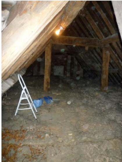
Intermediate truss looking in a westerly direction.
