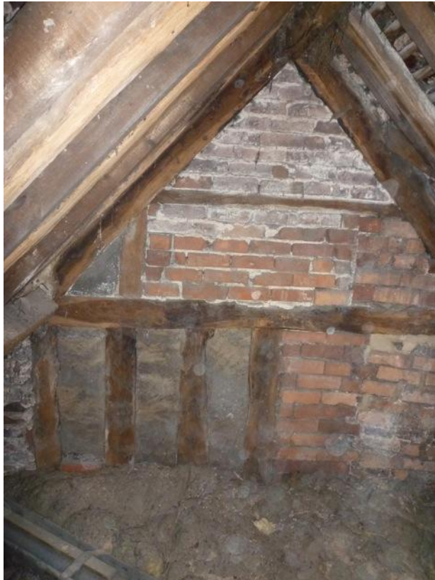
Roof space of south-east wing looking south.
