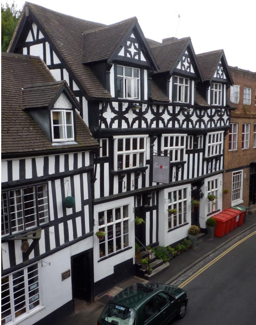
The Bailiff's House, 68-69 High Street, Bewdley, erected between 1607-10 with spurred quadrant braces to the front wall of the upper floor and gables. These braces are very similar to those used in the gables of 44 High Street, Droitwich.
