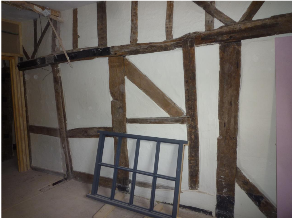
South side wall frame. The studs above the wall plate are secondary and were inserted when the brick wing in the foreground was added on to the south wall.
