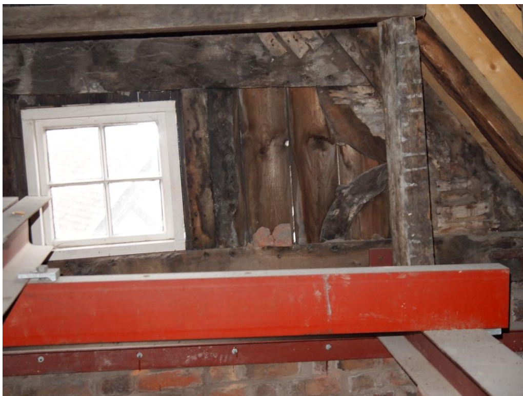
Decorative bracing below the collar of the High Street gables. (Photograph by courtesy of Paul Jones, LRPS.)
