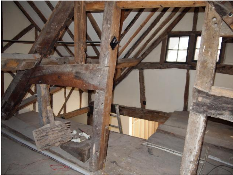
East-west range: detail of purlin housing in the central truss showing the split principal rafter. Photograph by courtesy of Paul Jones, LRPS.
