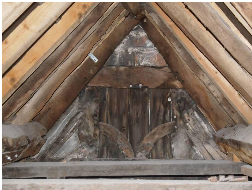
High Street frontage – timber-framed gable with decorative bracing visible above the collar internally, August 2014. (Photograph by courtesy of Paul Jones, LRPS.)
