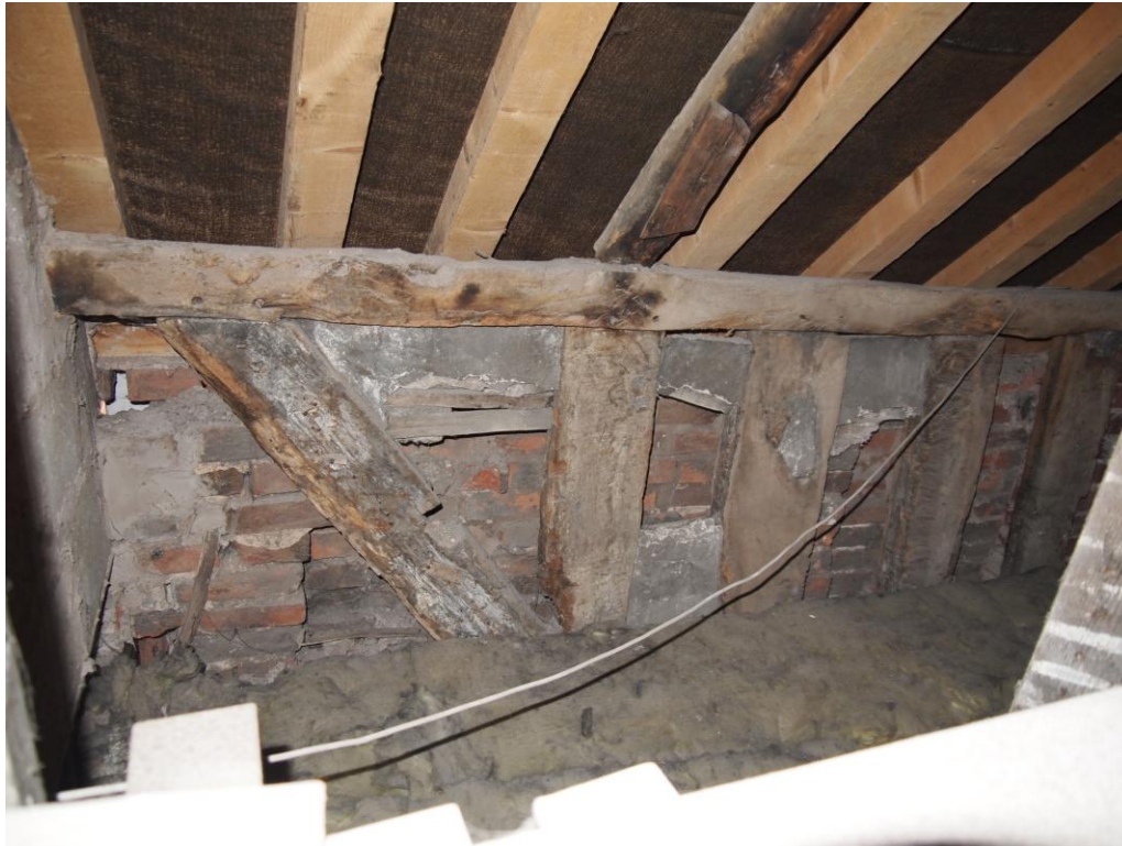
Close studding and brace in the side wall frame of the phase 2 extension visible internally at attic level. (Photograph by courtesy of Paul Jones, LRPS.)
