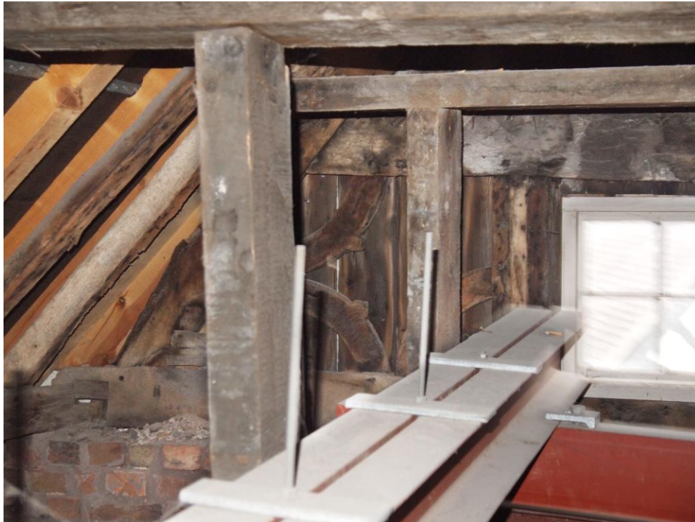
Decorative bracing below the collar in the attic of the High Street frontage, August 2014. (Photograph by courtesy of Paul Jones, LRPS.)
