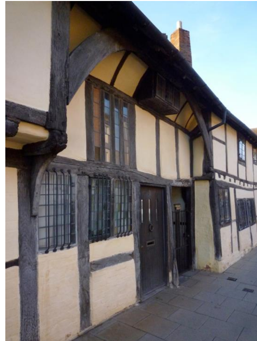
Mason's Court, Stratford-upon-Avon. The jettied bays either side the open hall and arch-braced wall plate with its coving in front of the hall window give an impression of what Droitwich's Wealden house would once have looked like.
