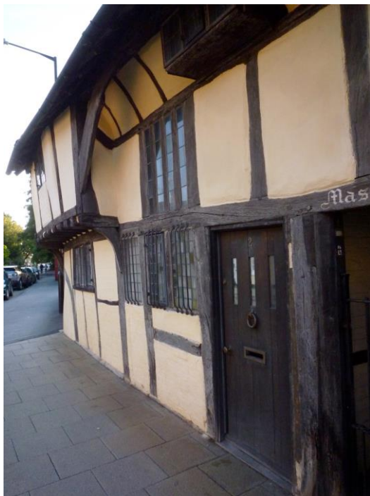
Mason's Court, Stratford-upon-Avon. The jettied bays either side the open hall and arch-braced wall plate with its coving in front of the hall window give an impression of what Droitwich's Wealden house would once have looked like.
