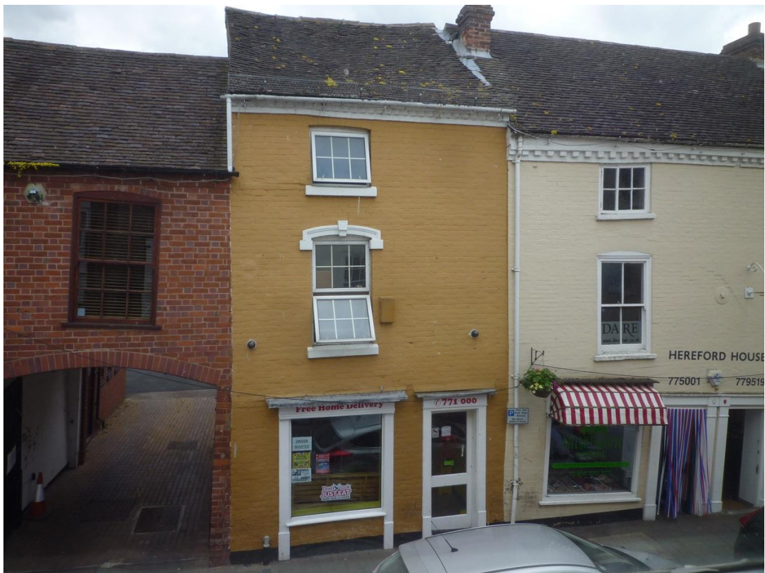
26 High Street – north or street elevation
