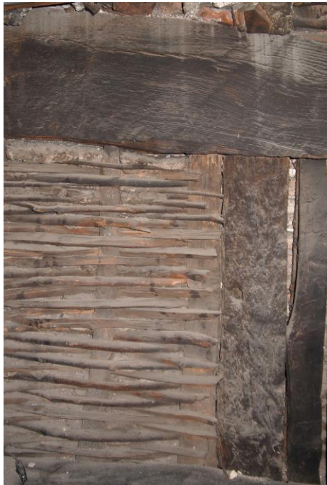
The west or upper face of part of T3 visible from within Spat's Coffee House at 22 High Street. The wattle infill woven round vertical staves is clearly visible. Photograph by courtesy of Paul Jones LRPS.
