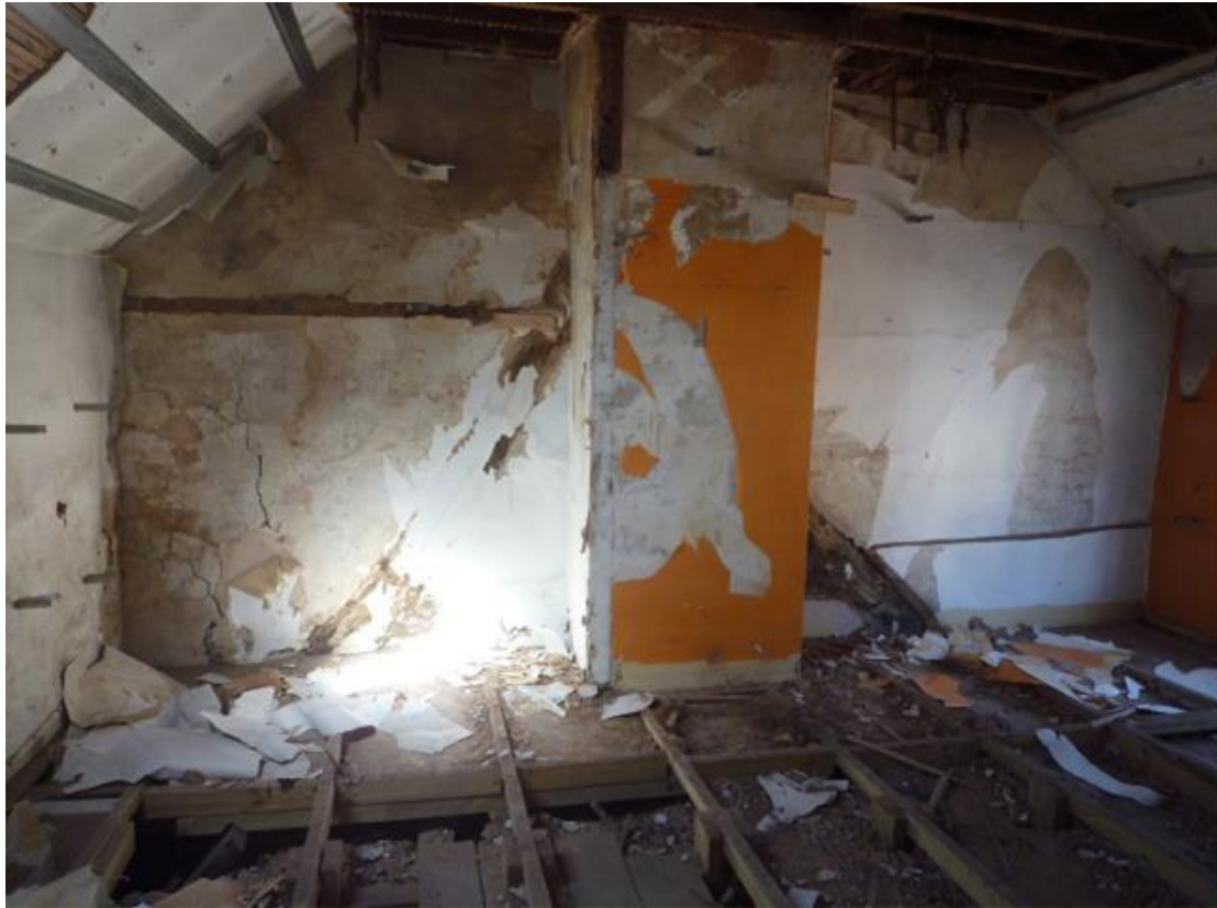
The upper part of the medieval roof truss T1 in the course of being uncovered against the west wall. The apex is hidden behind the later stack.
